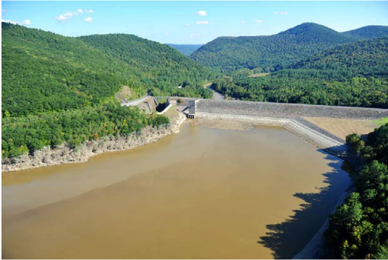
Suspended sediment collected at Townshend Dam, Vermont
