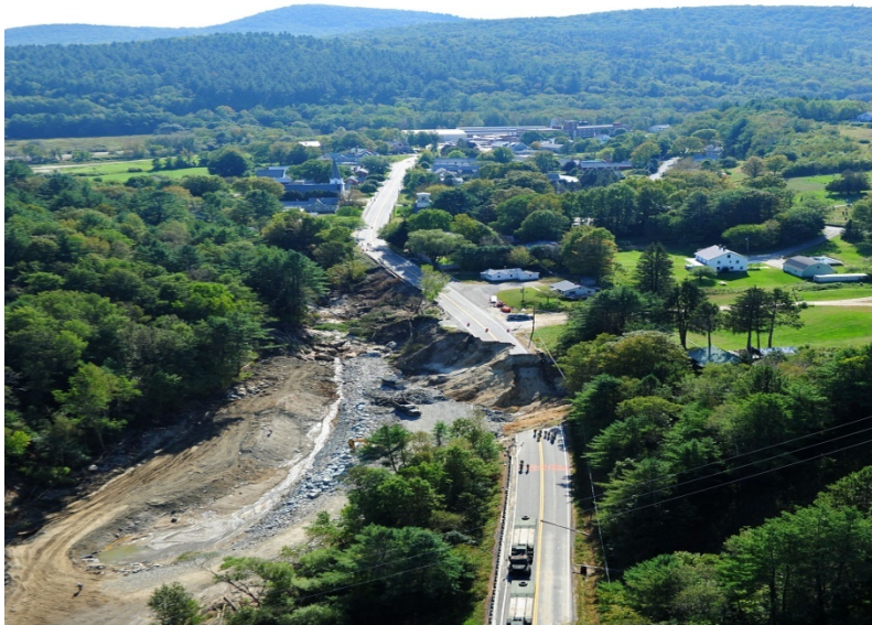
Highway damage in Vermont
