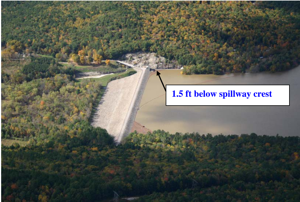
US Army Corps Surry Mountain Dam, Ashuelot River, Keene.
