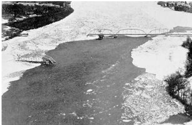
Ice Flows on the Kennebec River in Maine destroy highway bridge.
